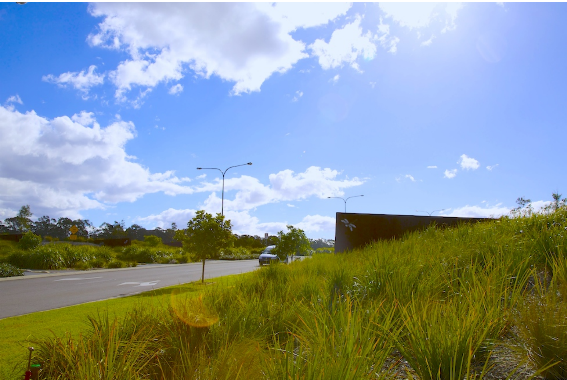
MASS PLANTED EMBANKMENTS
